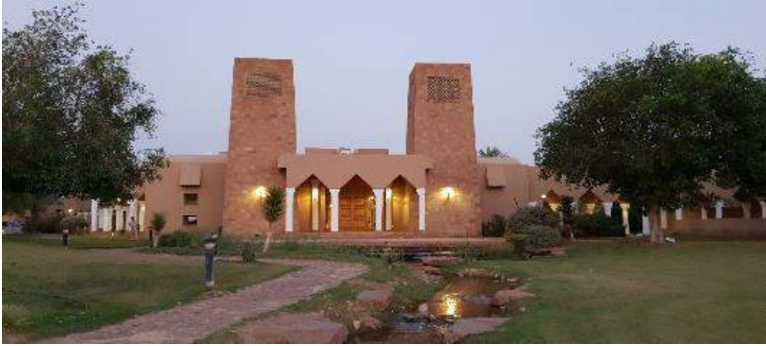
Figure 1: The main entrance of Dar Al-Rahmaniah library and the two PDEC towers
