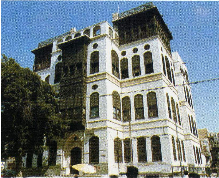
Figure (6) One of the finest examples of architecture in Old Jeddah, Nassif House, is a large merchant residence. The fretwork, mouldings, mashrabiyyah and fanlights have been preserved and restored to their original state. Source: Buchan (1986).
