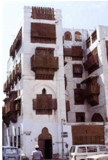
Figure (16) A four-storey house built out of coral in Jeddah with wooden rawasheen. Source: Al-Ban (2016).
