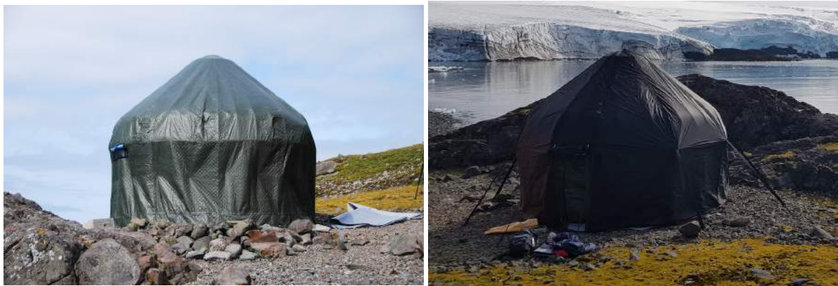
Figure 6. Left: First two layers of ORVEC put over the structure. Right: the external (third) layer of DYNEEMA.
