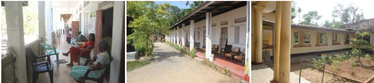
Figure 10. Colonnaded open verandas integrated with outdoor gardens and semi-outdoor courtyards
