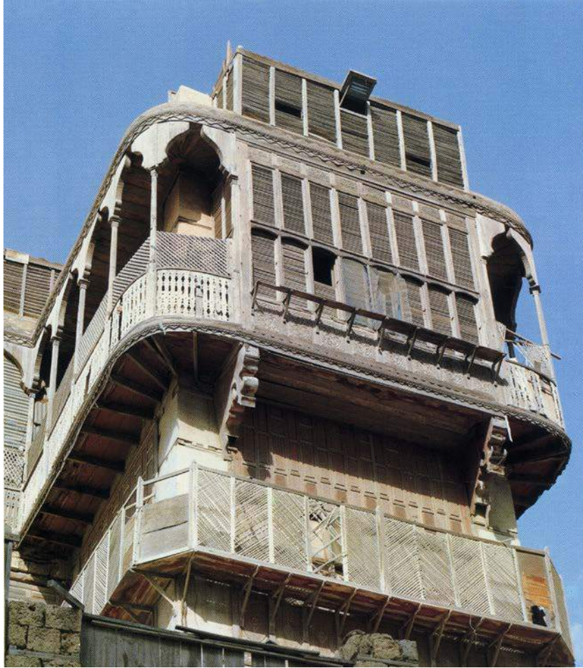
Figure 22 The projecting loggia of the large merchant house – Beit Al-Torki. Suspended six storeys above the street by a complex and carefully calculated sequence of cantilevers and crobels. This striking example of a chamber was where the whole family gathered together to enjoy cool onshore breezes. Source: Buchan (1986).
