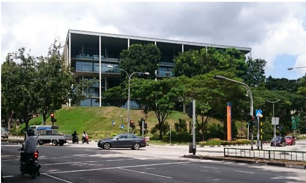
Figure 8. Image of the new Net Zero Energy School of Design at the National University of Singapore. The building is designed with Adaptive Comfort and supposedly the first of its kind in Asia. Image: Transsolar.
