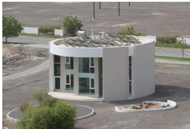
Figure 1. View from the north to the EcoHaus on the GUTech campus
