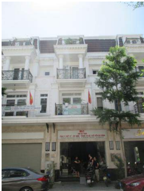
Figure 5: Building 3 view of Shophouse front
