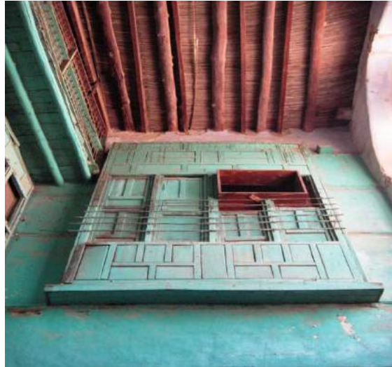
Figure (8) Timber roof of a typical traditional house Source: Kamal (2014)
