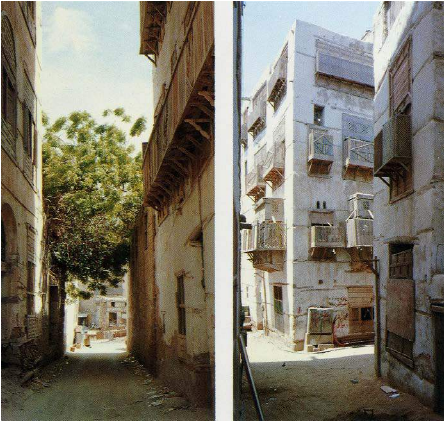
Figure (12) Tall houses catch the regular sea breezes and create upward drafts with their temperature differences. The overhanging open-louvered windows filter glare but allow air to circulate freely in the rooms. The streets are intentionally as narrow as possible to provide maximum shade. Source: Buchan (1986).
