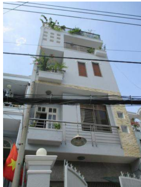
Figure 6: Building 4 view of front façade
