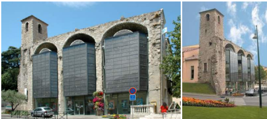
Figure 1. Integrated photovoltaics in the façade of historic building of Tourist Office in Alès (France) https://www.france-voyage.com/cities-towns/ales-9535/tourist-office-ales-5799.htm
