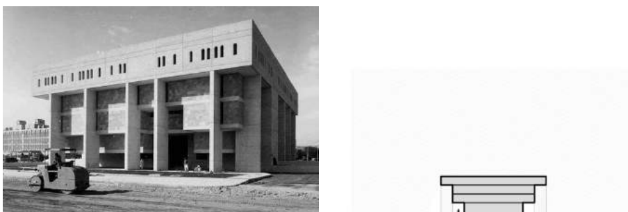
Figure 22. TAC: Kuwait Funds Building. 29.4°N, 48.0°E
