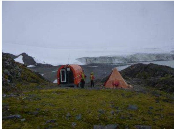
Figure 2. View of the Red Pod showing the metal frame sunk on legs into concrete foundations more than a meter deep.
