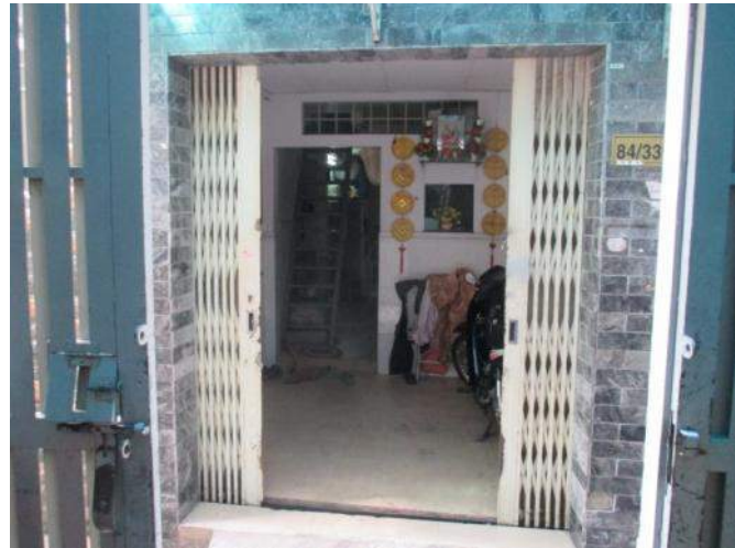
Figure 4: Building 2 view of entrance
