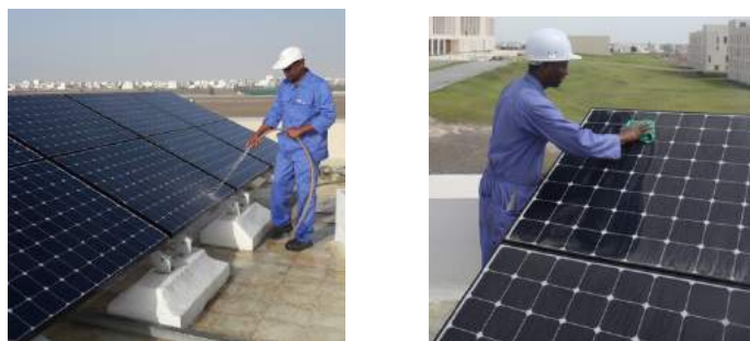
Figure 3. The maintenance team at work cleaning the PV modules
