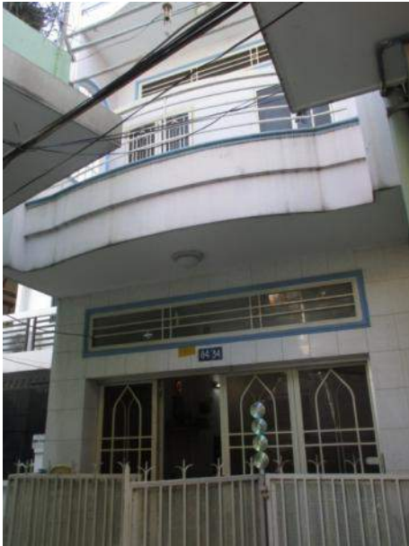
Figure 3: Building 1 view of entrance
