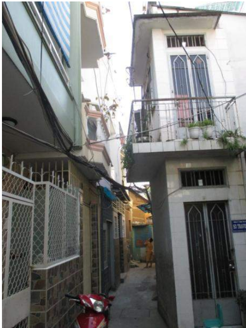
Figure 13: Poorly ventilated external space
