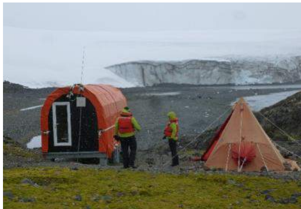
Figure 3. View of the Red Pod showing the metal frame sunk on legs into concrete foundations more than a meter deep.
