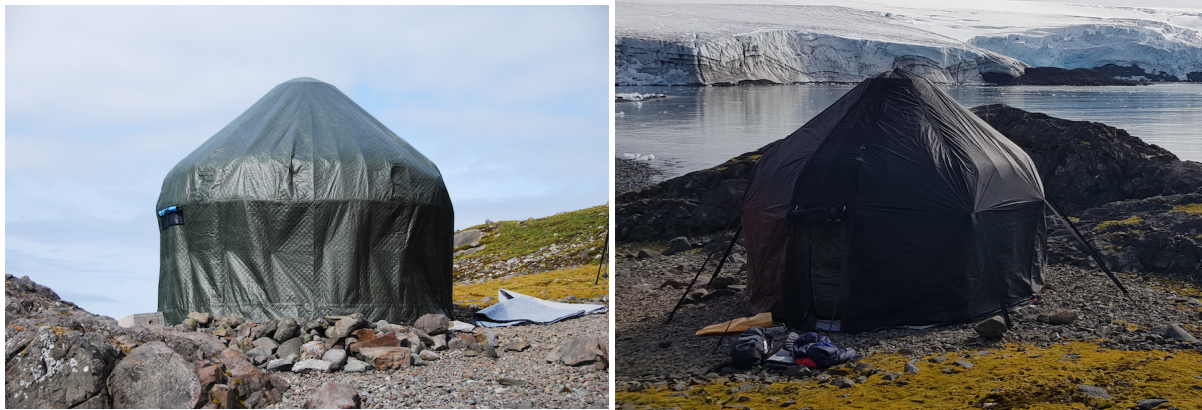
Figure 6. Left: First two layers of ORVEC put over the structure. Right: the external (third) layer of DYNEEMA.
