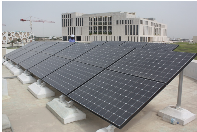
Figure 2. The roof-mounted PV system with ballasted racking
