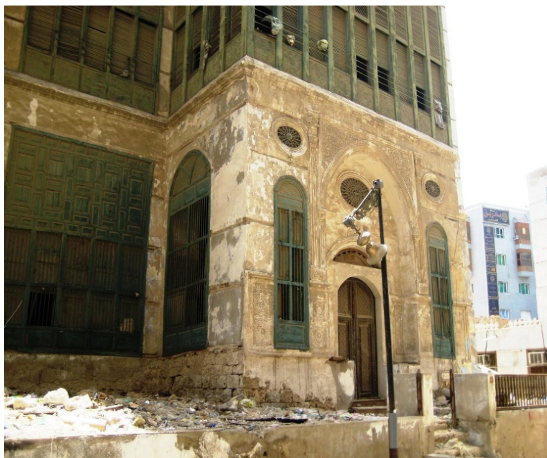
Figure (7) Ocean rock and coral stone load bearing construction Source: Kamal (2014)
