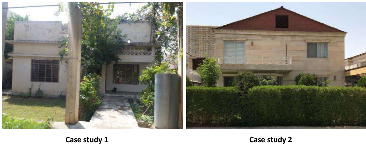
Figure 1 The front views of the examined houses (author)
