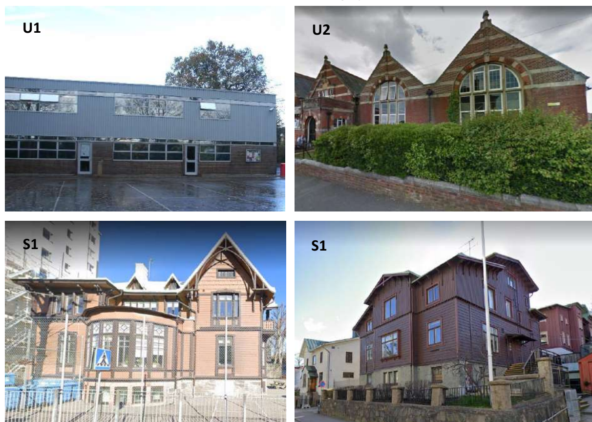
Figure 1. School buildings where the surveys took place. School S1 is housed in several buildings, two of which are shown here.
